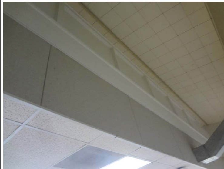
Photo -18 Building Number: 4 Ceiling condition within split classroom.
