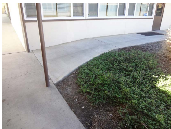
Photo -2 Building Number: 2 Non-compliant excessive slope condition at walkway.
