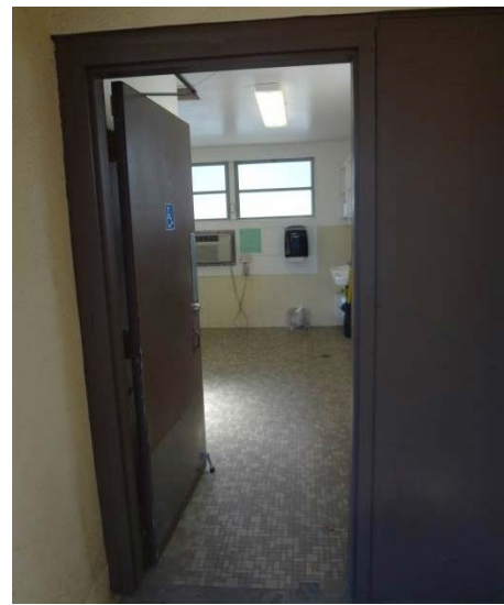
Photo -14 Building Number: 11 Narrow door threshold at Building 11.
