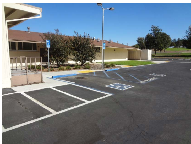
Photo -1 Building Number: 12 Accessible parking stall and detectable warning pavers.
