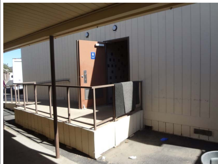
Photo -2 Building Number: 2 Non-compliant excessive slope condition at walkway.
