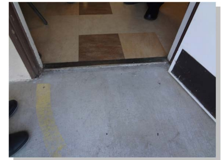
Photo -4 None of the thresholds have been updated to current accessibility standards.
